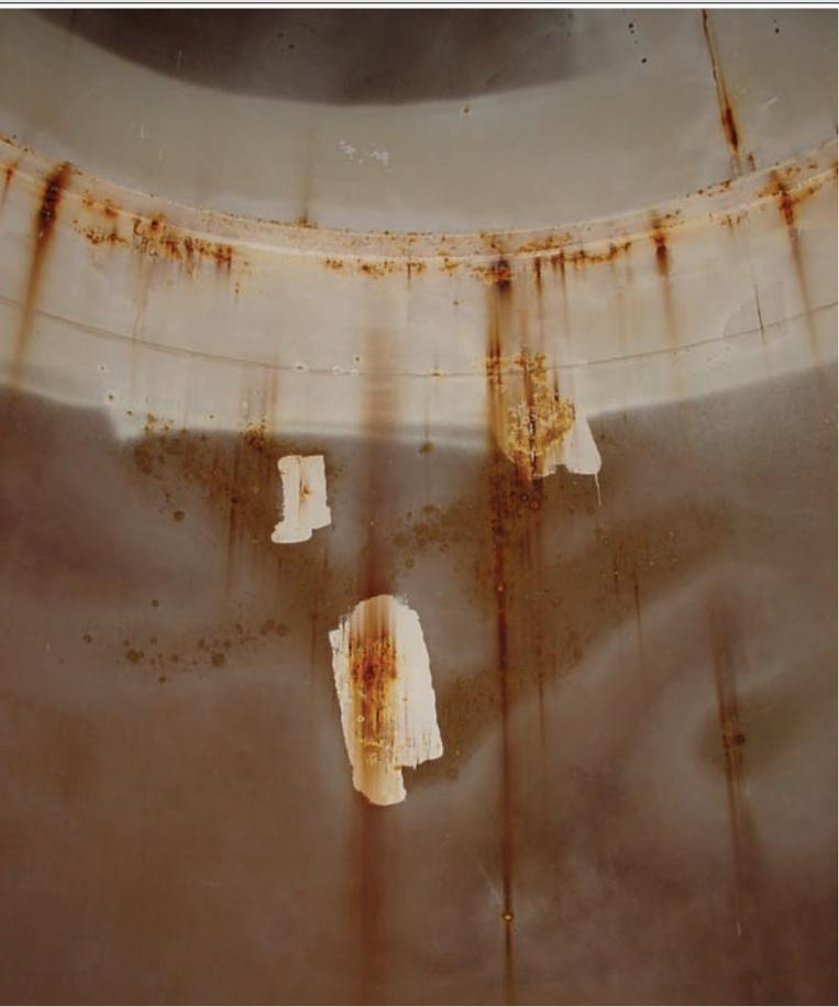
A botched paint touch-up job inside of this storage tank for a RWD in Kansas will require additional work.
