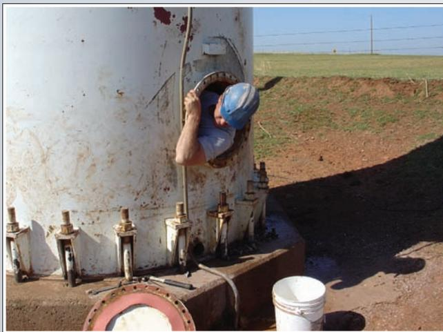
This manway is a tight fit for anyone. Adequate diameter of a manway is essential for subsequent operation and maintenance of water storage facilities.
