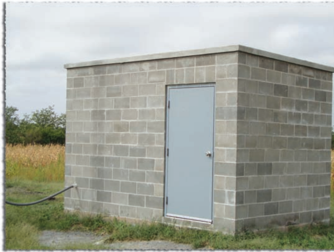
This new block structure was in place thirty-five days after the accident.
