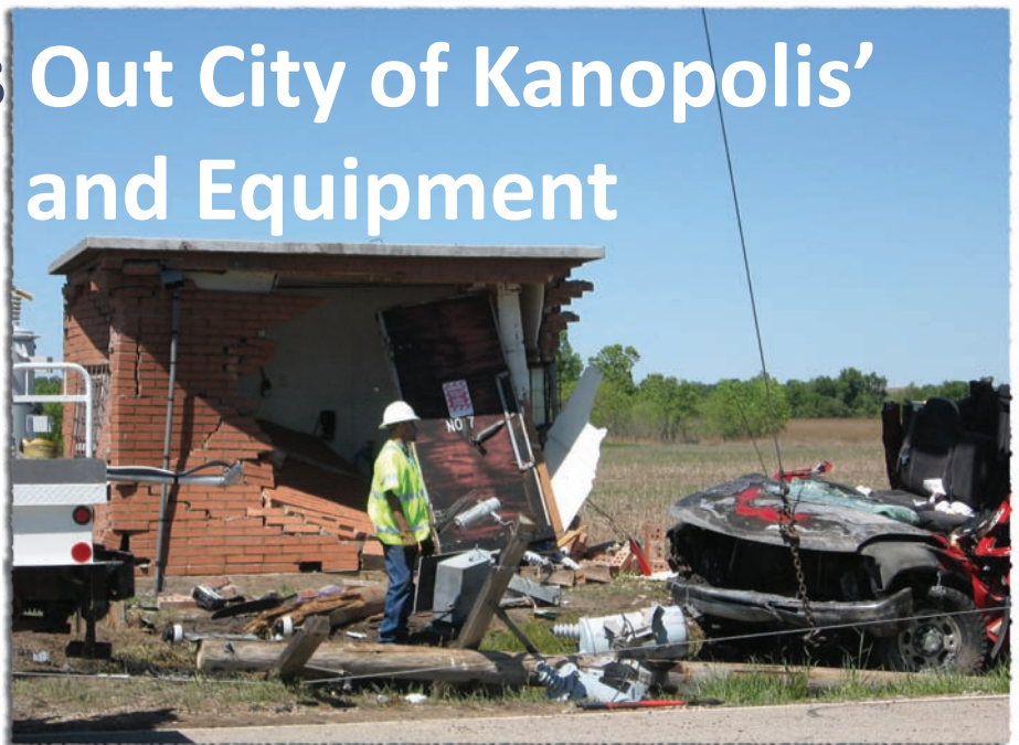
The city of Kanopolis' well house building, internal piping, chlorination system, telemetry controls and the power supply were destroyed by a pickup truck accident in May 2010.
