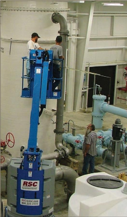
Workers install a seal in the piping for one of the two aeration towers in August 2010.
