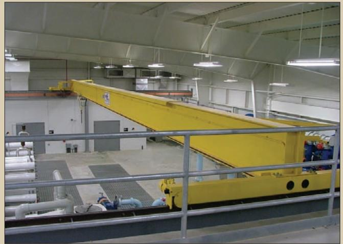
This photo shows the crane mounted on rails. The steel crane can be moved and positioned as needed to allow for removal of heavy equipment for maintenance.
