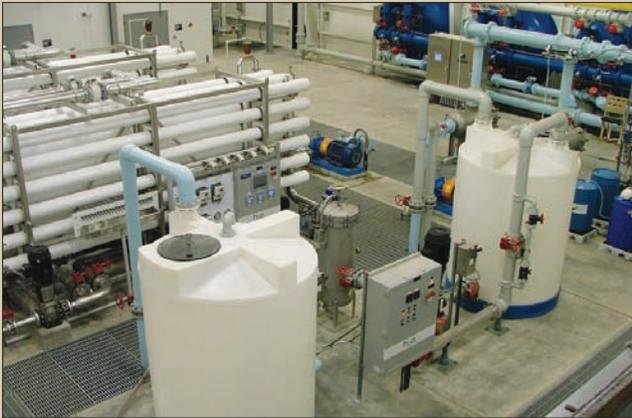
The plant layout can be visualized from the mezzanine area. The two tanks in the foreground are used in the clean-in-place process for cleaning the membranes. Also shown are the membranes on the left, and greensand filters in the background.
