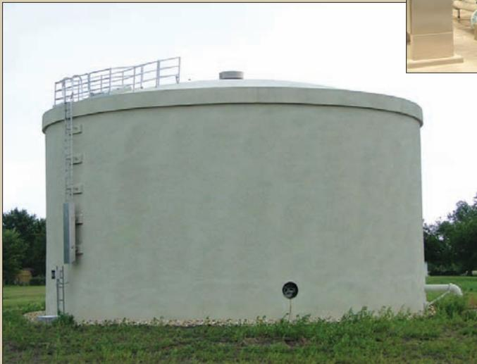
This photo shows the 0.500 MG wire-wound pre-stressed concrete storage tank that stores finished water. Water from this tank is pumped to the distribution system as needed. Natgun Corporation with corporate offices in Wakefield, MA, provided this tank.
