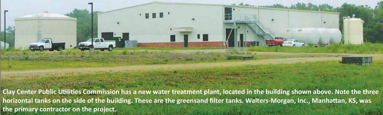
Clay Center Public Utilities Commission has a new water treatment plant, located in the building shown above. Note the three horizontal tanks on the side of the building. These are the greensand filter tanks. Walters-Morgan, Inc., Manhattan, KS, was the primary contractor on the project.
