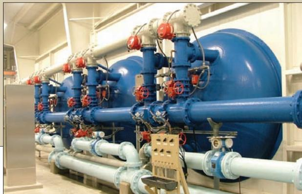
An "end view" of the three-greensand filters, the first treatment unit. Most of the tank extends outside the plant building.
