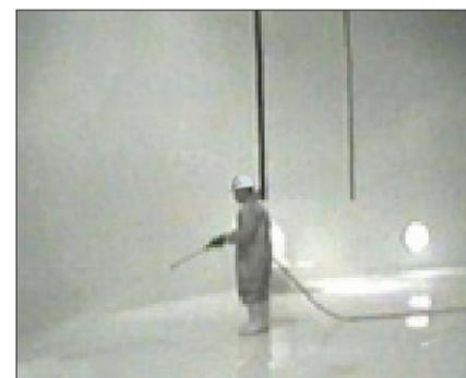
**Figure 4: Distribution tank after NSF 60 chemical cleaning to remove bio-film.**
