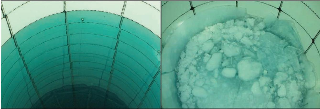
Figure 8: Photographs of the interior of the same tank with and without mixing and ice formation.
