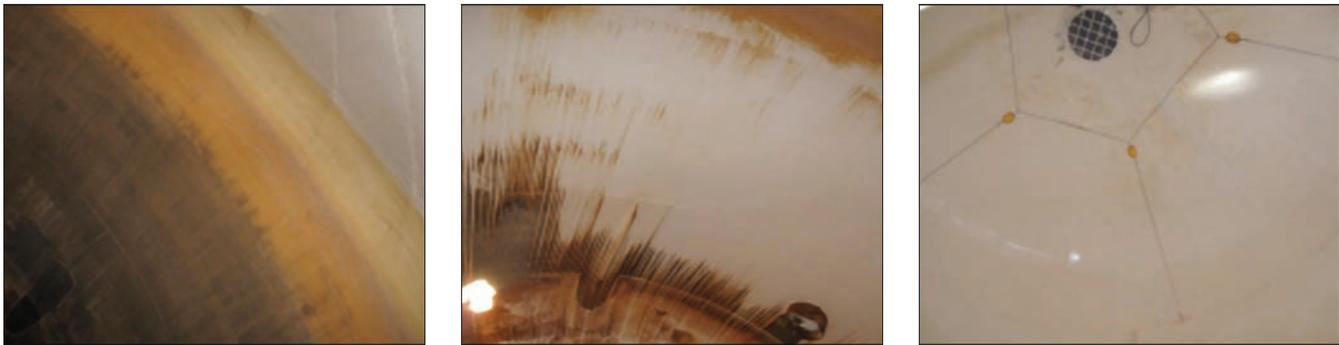
Figure 5: Before, during and after chemical cleaning of a tank interior to remove bio-film and deposits
