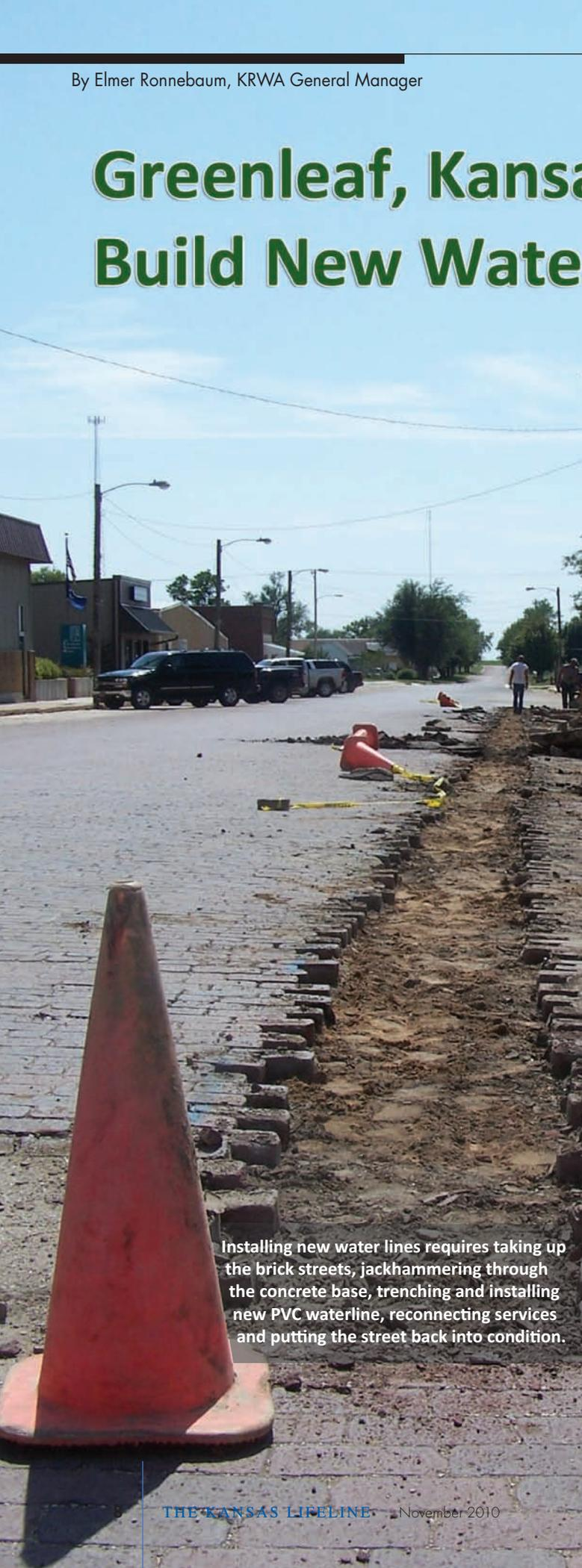
Installing new water lines requires taking up the brick streets, jackhammering through the concrete base, trenching and installing new PVC waterline, reconnecting services and putting the street back into condition.
