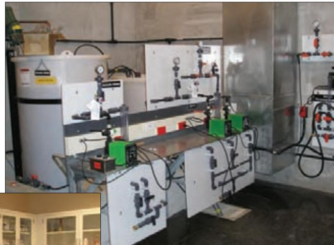
**Above: The plant's chemical room administers coagulants, polymer, ammonium sulfate, and a phosphate.**
