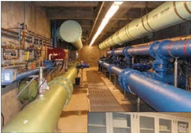
**Pipe chase connecting the solids contact basins to the filters**
