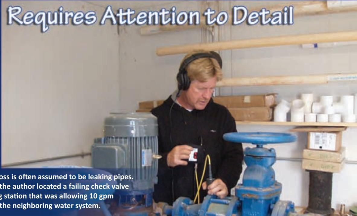
High water loss is often assumed to be leaking pipes. In this case, the author located a failing check valve in a pumping station that was allowing 10 gpm backflow to the neighboring water system.
