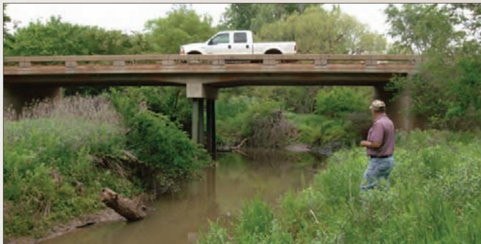
**Harper County RWD 4 Operator Jim Coady surveys the location where a 30-gpm leak was located on this crossing. Replacement will involve a directional bore of approximately 250 feet.**
