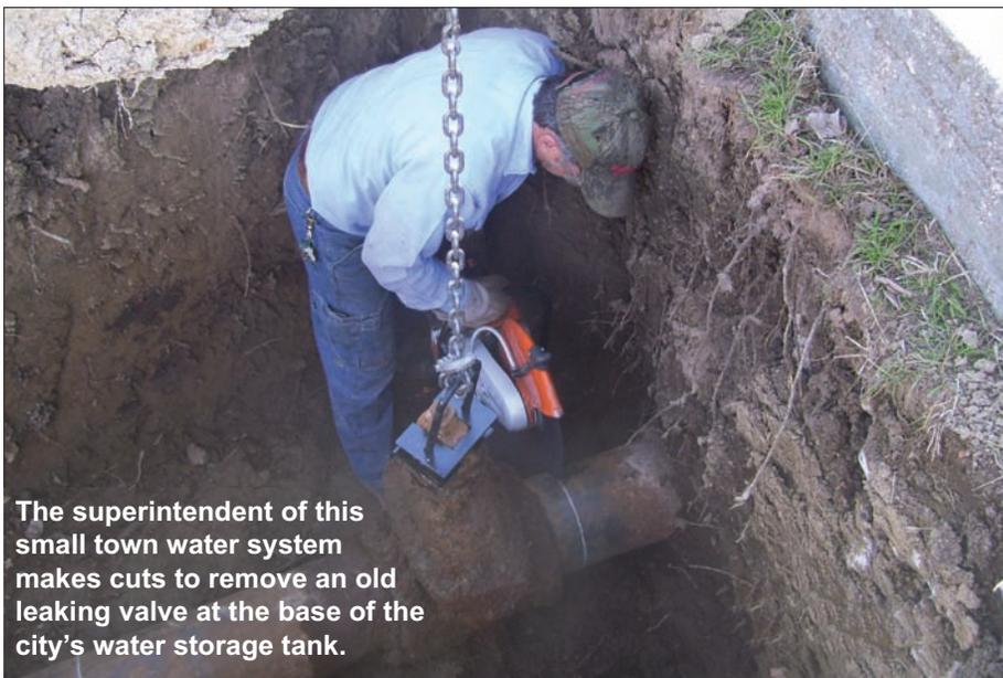
The superintendent of this small town water system makes cuts to remove an old leaking valve at the base of the city's water storage tank.
