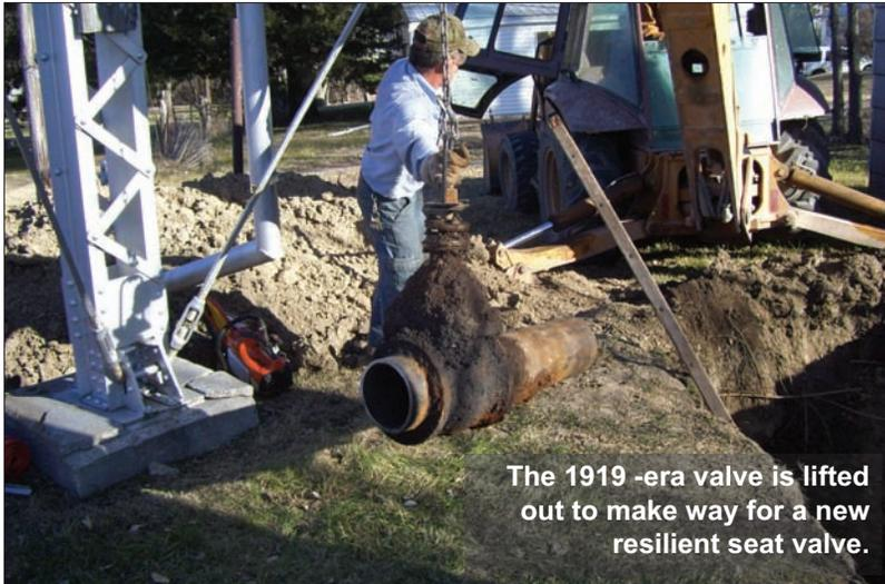
The 1919-era valve is lifted out to make way for a new resilient seat valve.
