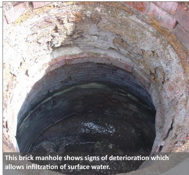
This brick manhole shows signs of deterioration which allows infiltration of surface water.
