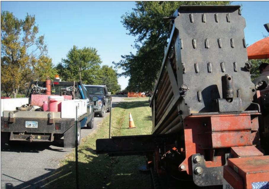
Duling Construction Company, Inc., Wichita, was contracted to install new waterlines in Udall. At a cost of nearly \$927,000, nearly all lines were directional bored.
