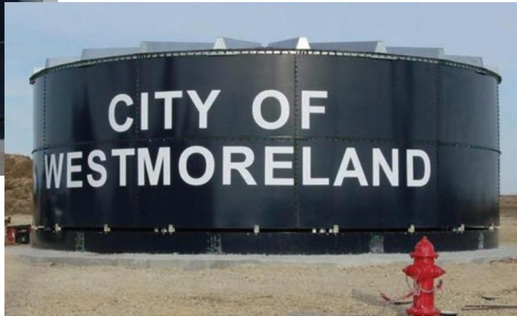
out of the tank to prevent loss of chlorine residuals. This project also included 2,800 feet of 8-inch PVC pipe to connect the new tank to the existing distribution system. Plans are to have the tank in service by early spring 2010, as construction has been delayed due to weather. The project also included teardown and removal of the old steel tank.
