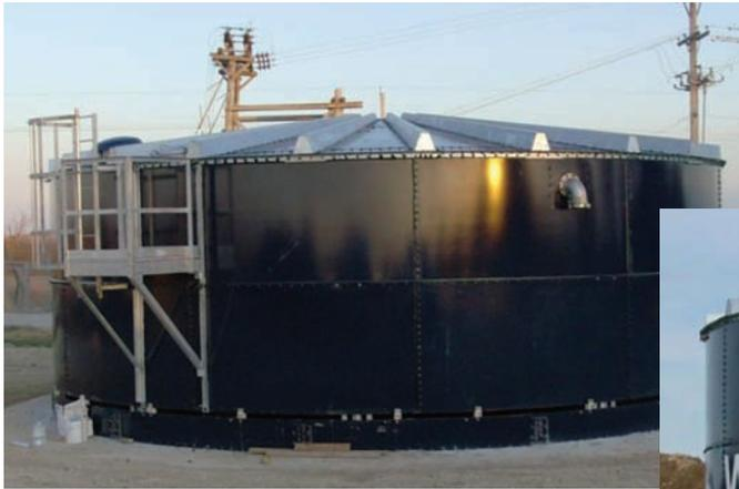
These photos show the front and back sides of the tank as construction begins with the first two rings. When completed, 13 rings, each 54 inches in height, will be needed to reach a height of 61 feet. The other photo shows the overflow and a safety cage that will be seen from the side opposite the majority of the city.
