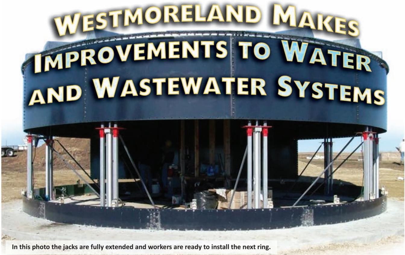
In this photo the jacks are fully extended and workers are ready to install the next ring.
