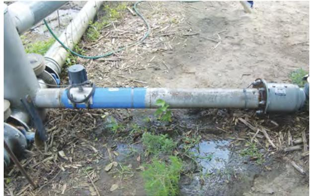
The typical installation of an irrigation flow meter is shown in this photo.
