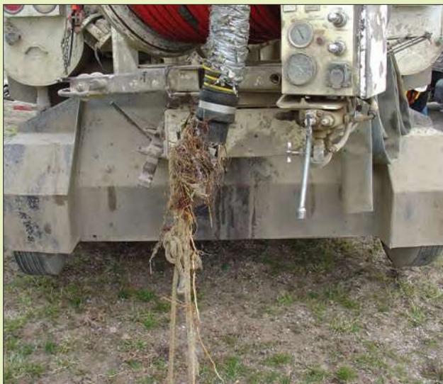
This photo shows a small bundle of tree roots that were dislodged during a cleaning project and which subsequently created a blockage in a sanitary sewer line.
