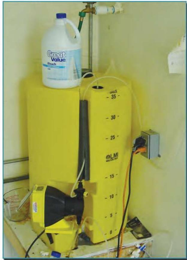
This photo shows the rechlorination system at Atchison Cons. RWD 5. The system adds six percent bleach to increase the chlorine residual. Ammonia is also added.
