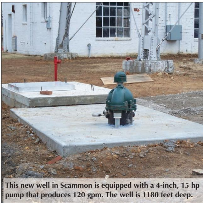
This new well in Scammon is equipped with a 4-inch, 15 hp pump that produces 120 gpm. The well is 1180 feet deep.
