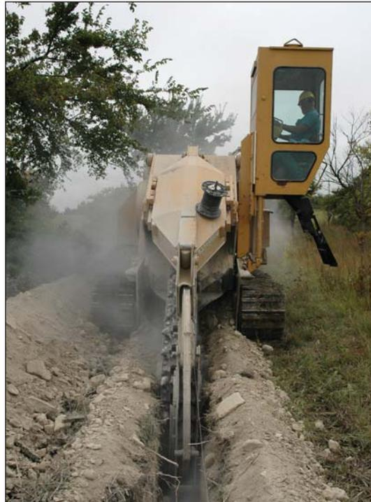
*This photo of a trencher digging through rocky terrain was taken during the installation of a rural water district funded by USDA Rural Development.*
