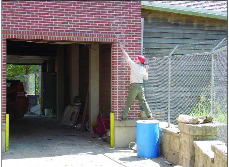
*KRWA consultant Pat McCool stretches to point to the height the flood waters reached at the Fredonia Water Treatment Plant. The building shown houses the water lab, office, and raw water pumps, all of which were submerged under approximately 10 feet of flood water.*
