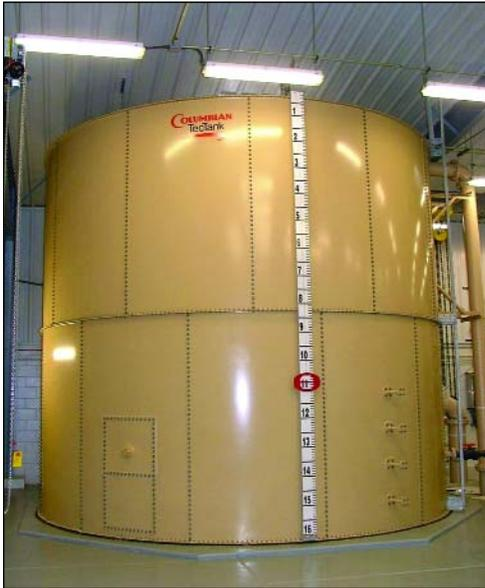
*This tank is being used as the filter backwash holding tank.*
