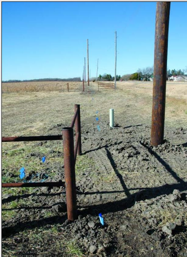
*The Sedgwick County Rural Water District No. 3 water line, marked with blue flags, lies between power poles and a private fence. A communications line either parallels or crosses the water line at the light green can in the center of the picture. The district's water line took numerous hits during a project to relocate power and telephone utility for road widening. Because of legal considerations the district was not able to move the line before other utilities started construction.*
