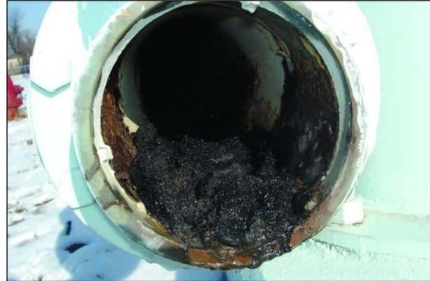
**Above right:** An abundance of sand-blasting material was found at this system inside of a water tank overflow pipe.
