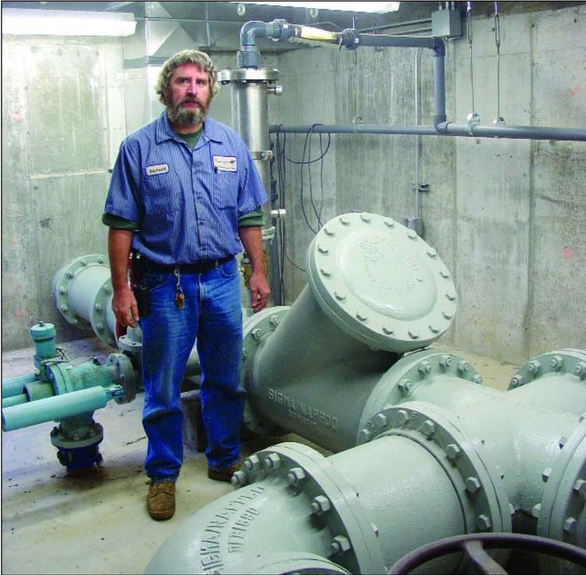
Marysville utility employee, Richard Kyle, stands next to the 16-inch wye used to introduce the poly pig for cleaning the Marysville force main. Valves allow the force main to be shut off so no back flow will come from the force main.
