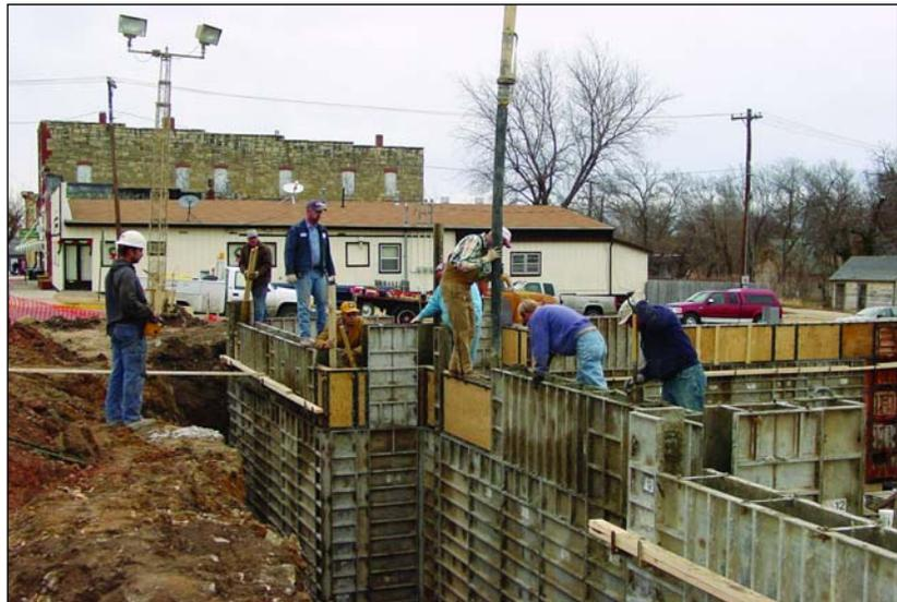
This photo shows a wall pour in progress. Many different fasteners are required to hold forms together in order to pour a concrete wall.
