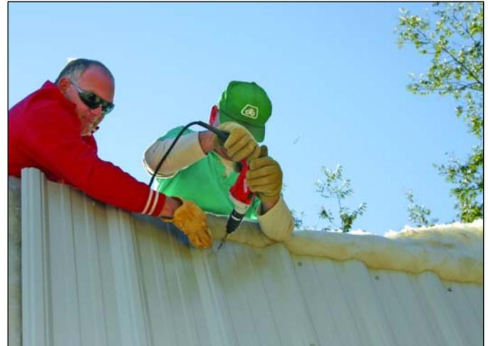
Self-tapping screws are commonly used for metal buildings to ensure penetration into the main frame of the building and solid placement.
