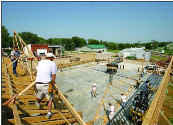
Workers begin to stand the trusses on September 5. A severe wind storm made this part of the project double work as the previous set of trusses were blown down. Luckily, workers were just finishing; no one was injured.
