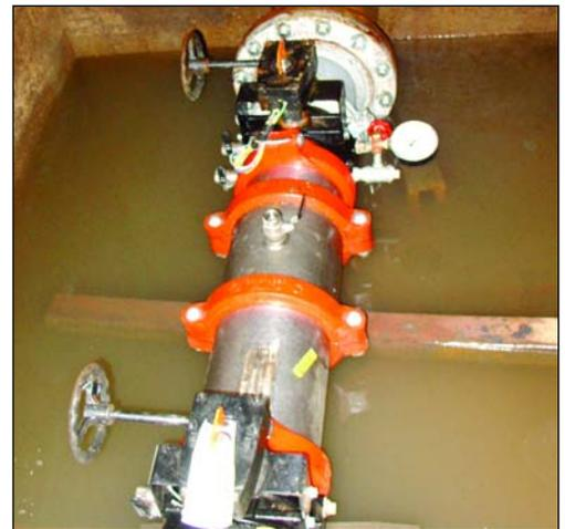
industry is now also protected with a proper, testable double-check valve (DCV) assembly. The city and the industry should both be commended for their efforts in taking positive action to protect the city's water supply and the water supply for employees at the industry
