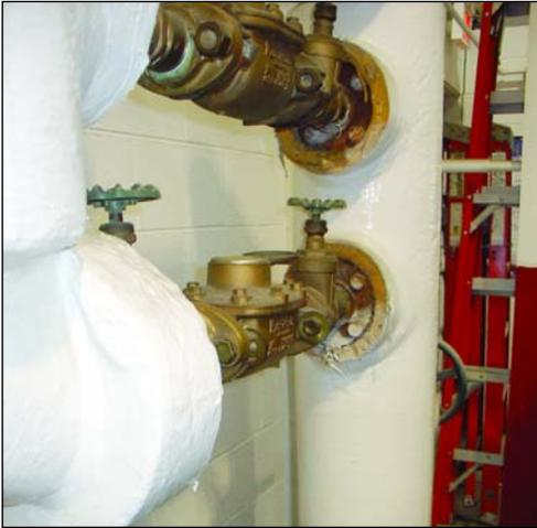
**Left:** The main water supply line to an industry without a backflow prevention device.
