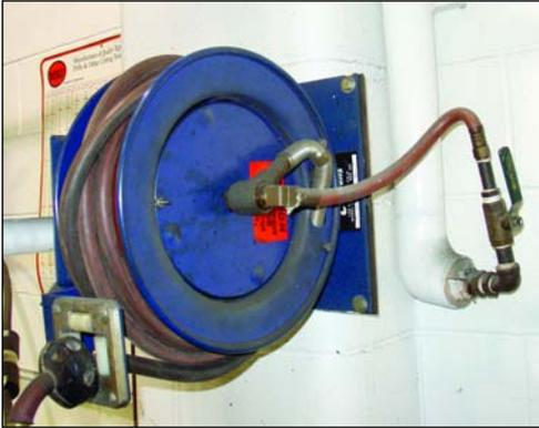
**Left:** A hose connected to a water line without a backflow prevention device.
