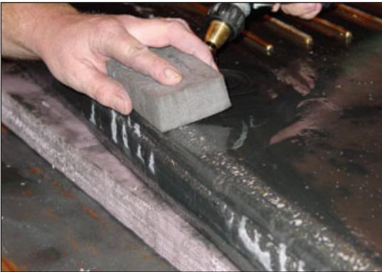
*Shane applies a little elbow grease in the knock-down and polishing process that exposes the aggregate (look on the rounded edge) and smooths the counter top's finish.*
