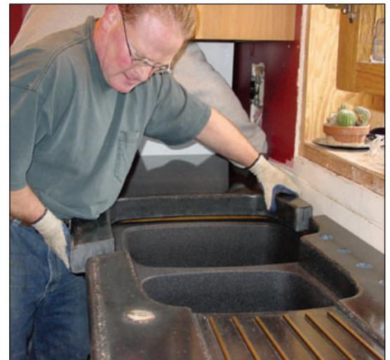
*Shane jogs the second sink section into place. Notice the narrow points around the sink that needed the 3/8 in. rebar reinforcement for extra strength. A break certainly isn't needed at this point.*
