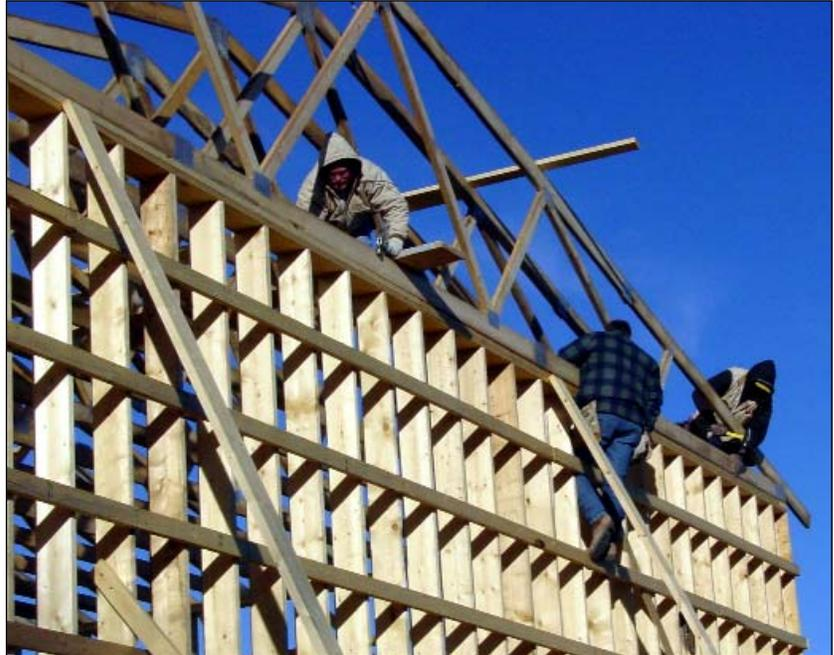
*Together up high, workers on the KAN STEP fire station project at McFarland, Kan. communicate to properly place and nail trussed rafters.*
