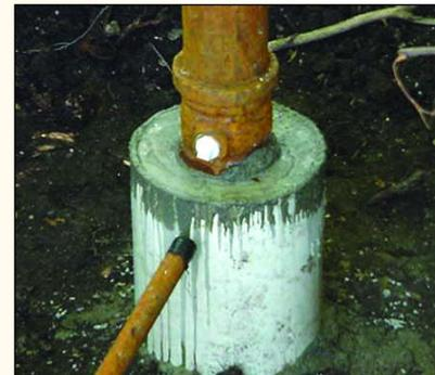
The problem was remedied after the well was cleaned and an eight-inch PVC casing was placed on the outside of the original well casing and grouted to prevent any further incursion of roots.
