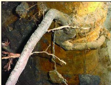
Above, a medium-sized root is wrapped around the 5-inch well casing. Because this casing had only been spot welded at a section joint (see below), the roots were able to grow into the well. The plug of tree roots was removed from the well.
