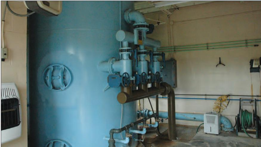
The city operates a battery of wells in addition to purchasing water from Jefferson County RWD No. 13. The city treats its well water supply through this single vessel filter to remove iron and manganese.
