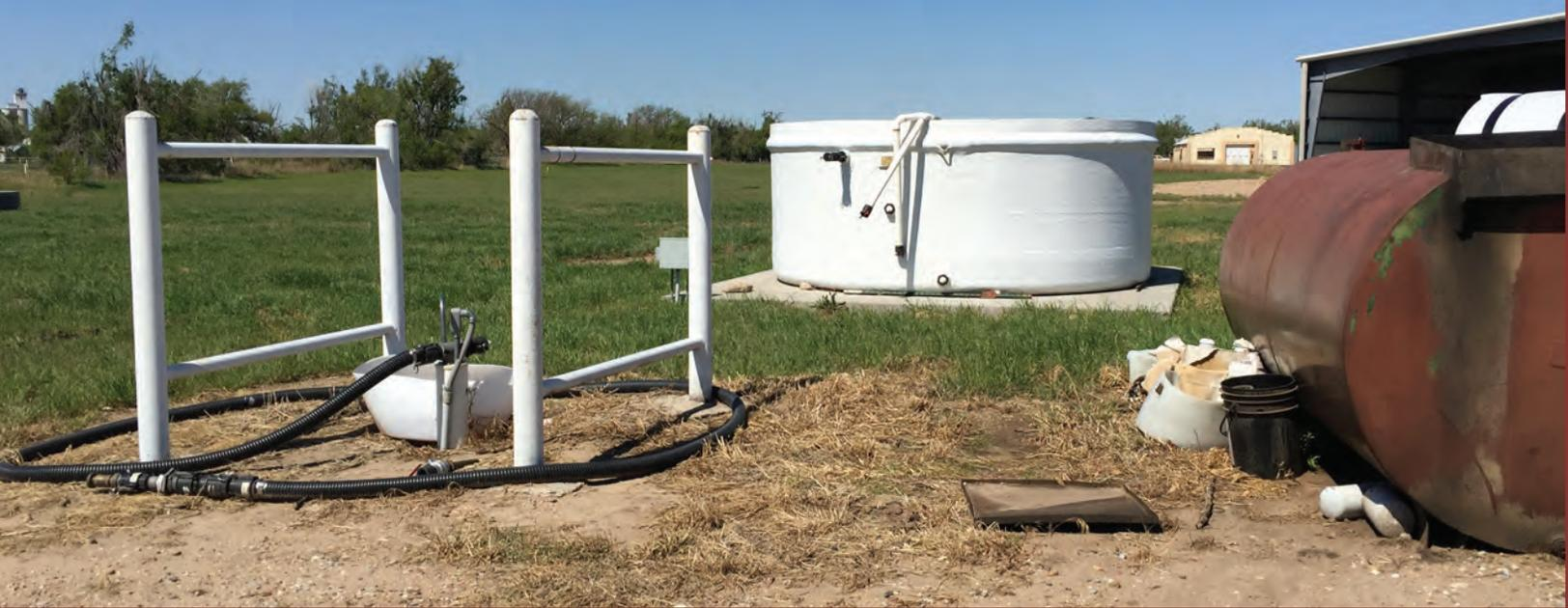
This well on the left side of the photo is protected from vehicle collisions with steel piping, but not from leaks or spills from the nearby storage tank, chemical totes, and un-empty trailer mounted tanks. The steel tank on the right appears to store used motor oil based on the presence of used oil filters on the ground.
