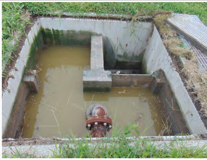
**Changes in water elevation can be detected and can indicate when a blockage has been contributing to bypasses to the other cell.**
