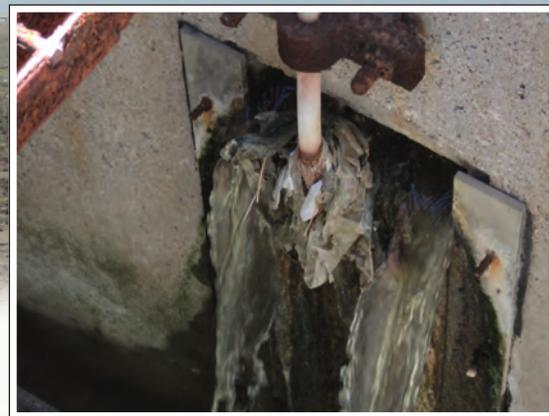
Debris on the slide gate in a structure at a lagoon can also cause bypasses.
