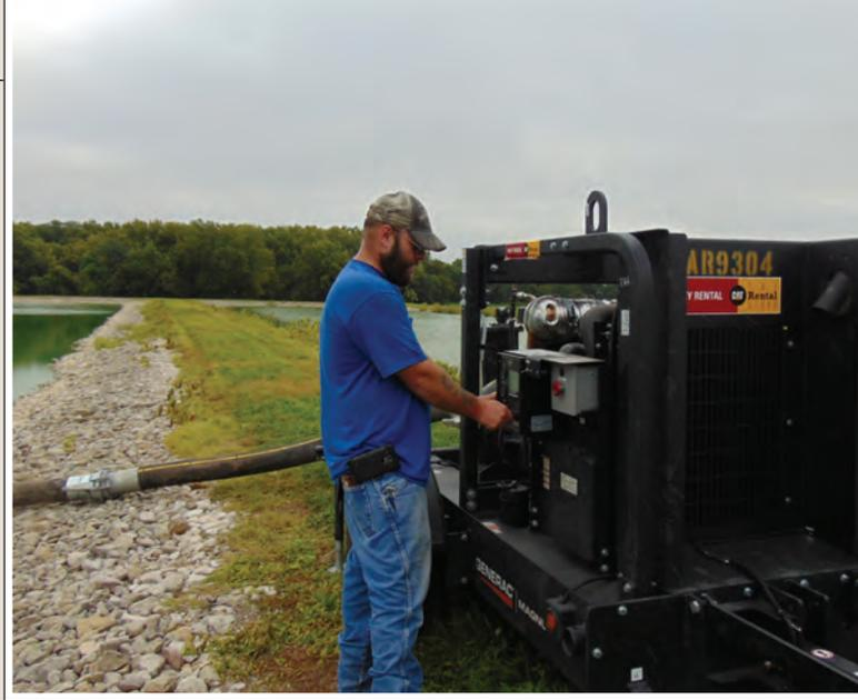
**Keith Murphy, operator at McFarland, starts the pump to bypass Cell 1 to lower the water level to allow for removal of debris and the turtle guard.**
