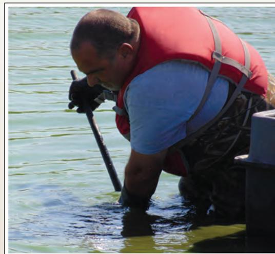
KRWA Wastewater Tech Charlie Schwindamann uses a large pry bar to remove the turtle guard and debris from the influent pipe to the primary cell.
