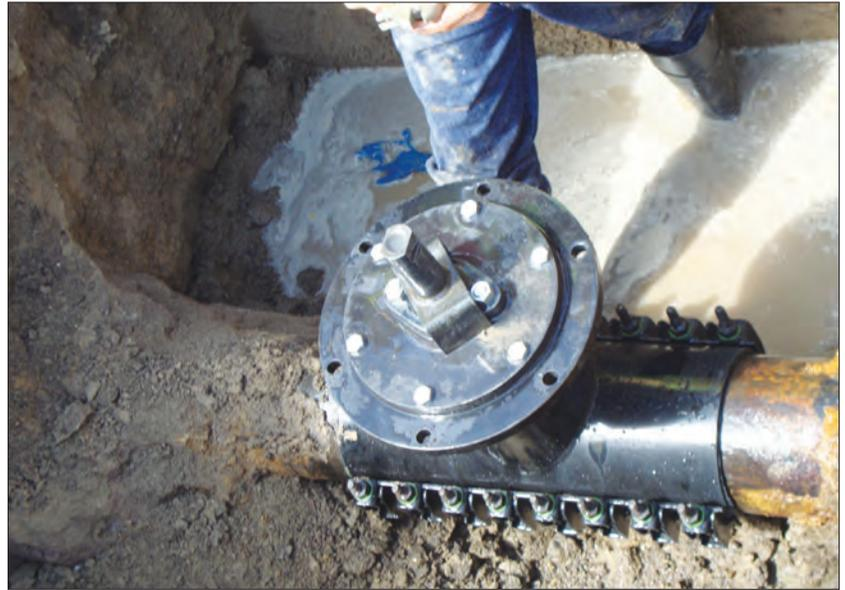
This close up shows a new 8-inch valve insertion. Most of the Smith Center's distribution system is cast iron.
