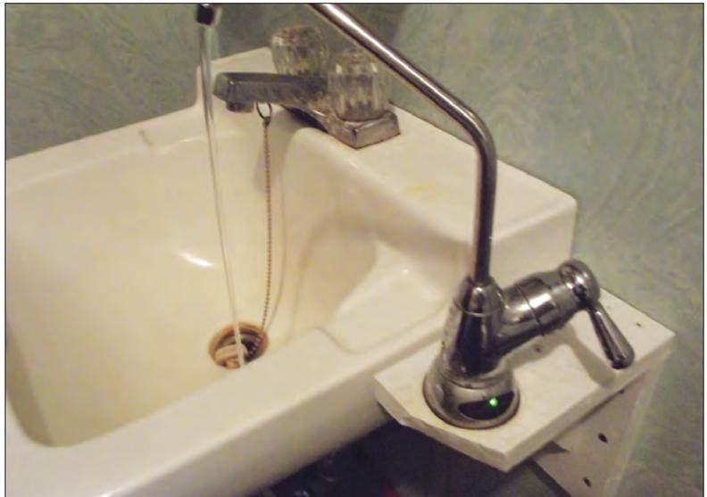
This separate faucet provides treated water. The green light indicates that the system is working properly. The monitoring system would show a red light instead if the system needs to be checked. Each home has one such faucet that provides the treated drinking water.
