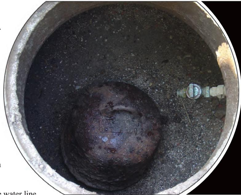
Flush tanks, such as that shown above, are no longer installed in sewer lines. These are potential direct cross connections. For those that remain in some municipal wastewater system, the water lines should be removed from them to make sure there is no possibility of contamination in case of a water line break and there is a sewer back up at same time!
