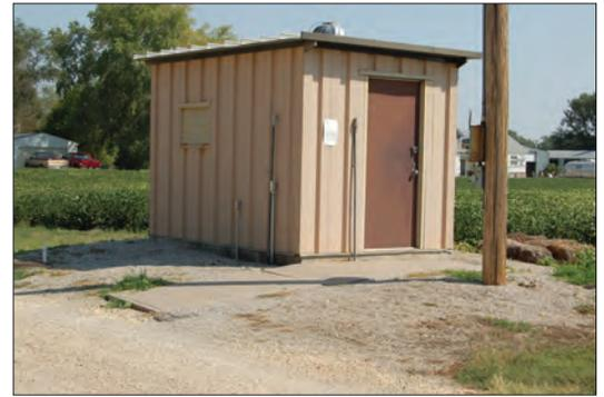
This structure is the wellhouse for Well No. 6 and the chlorination building.
