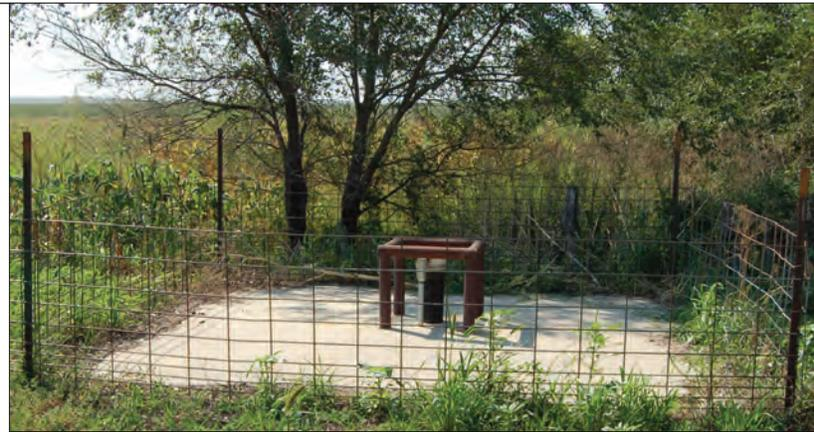
**Well No. 7 is protected by welded steel pipe, fencing and a large concrete pad. Additional protection measures for wells 1, 6 and 7 will be identified and implemented.**
