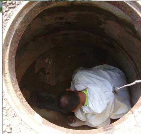
**A worker from Mayer Specialty works to line a manhole with polyurethane coating.**
