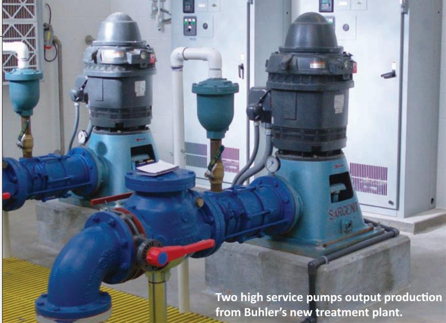
Two high service pumps output production from Buhler's new treatment plant.
