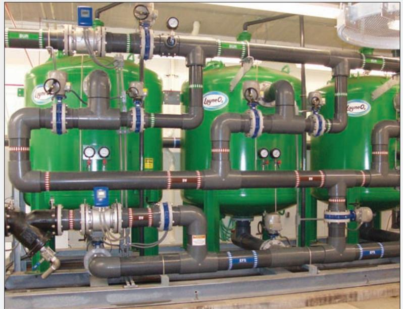
This photo shows the filter system by LayneOx; it removes iron and manganese and arsenic.
