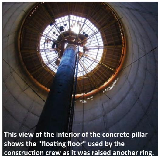
This view of the interior of the concrete pillar shows the "floating floor" used by the construction crew as it was raised another ring.
