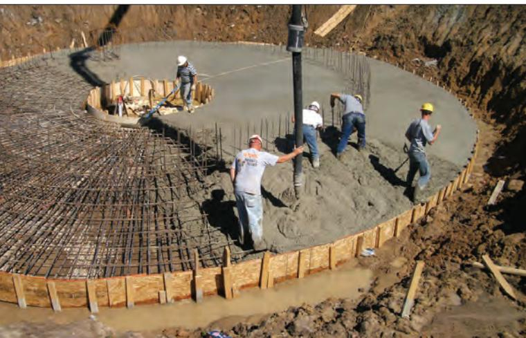
Concrete is being placed for the base of the new storage tank.
