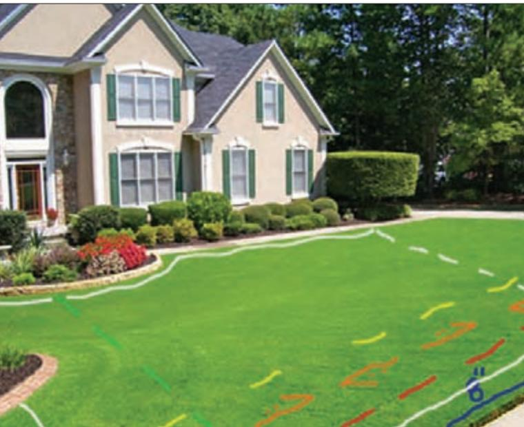
At a location where proper methods are employed, an excavation area is identified with white lines or flags and all utilities are located within that area. This photo shows the intended zone of excavation, green for a sewer line, yellow for gas, orange for fiber optic and blue for water.
