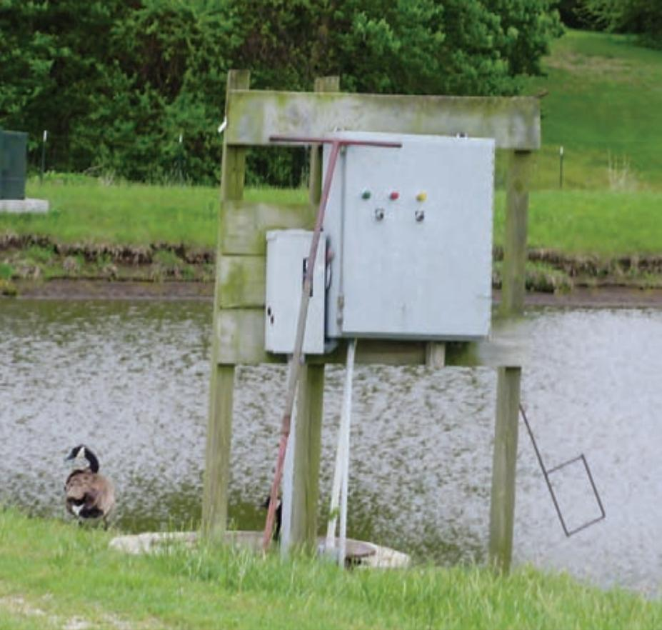
This pump station for a typical lagoon irrigation system is located next to the final cell. A pipe from that cell connects to the pump station wet well. The wet well is equipped with a submersible pump that pumps wastewater to be irrigated to a nearby sprinkler system. Such systems are often also equipped with timers that allow running several cycles each day. This helps ensure runoff is not a problem. This pump station was also doubling as a nesting site for a pair of Canada Geese.
