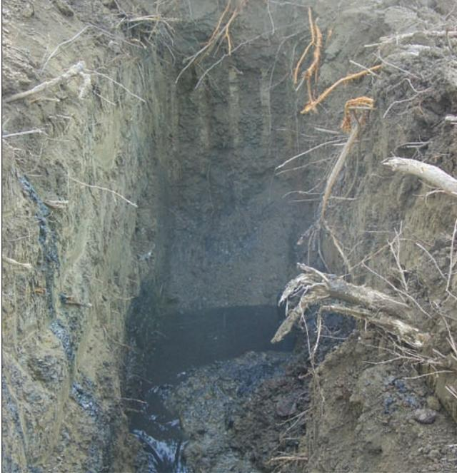
**This photo shows excavation of an 8-inch sewer main that had a blockage; a sewer machine could not clear the blockage. Tree roots had penetrated this sewer line, resulting in a complete blockage. The blockage was removed, reestablishing flow. This line was replaced as soon as the city obtained materials.**
