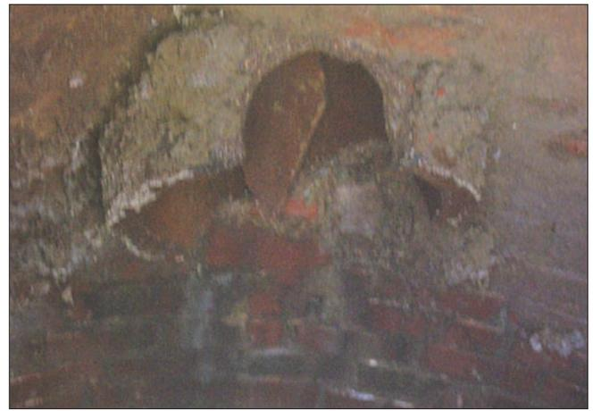
**A broken piece of clay pipe can be seen in the inlet pipe.**
