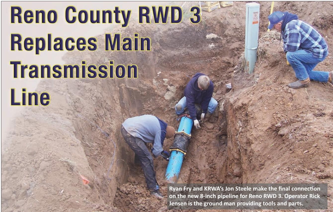
Ryan Fry and KRWA's Jon Steele make the final connection on the new 8-inch pipeline for Reno RWD 3. Operator Rick Jensen is the ground man providing tools and parts.
